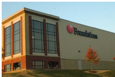
High Resolution Photo of the new Foundations ® Children's Products facility in Medina, Ohio.
